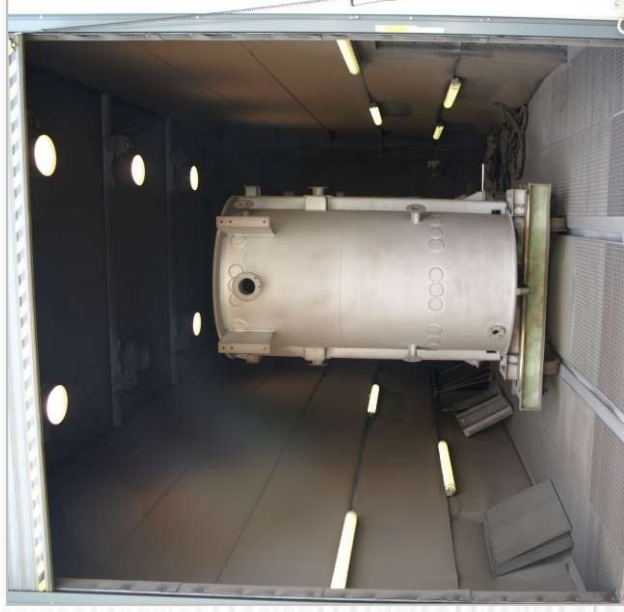
Transformer tank in blast chamber
